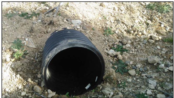
Newly installed culvert.
