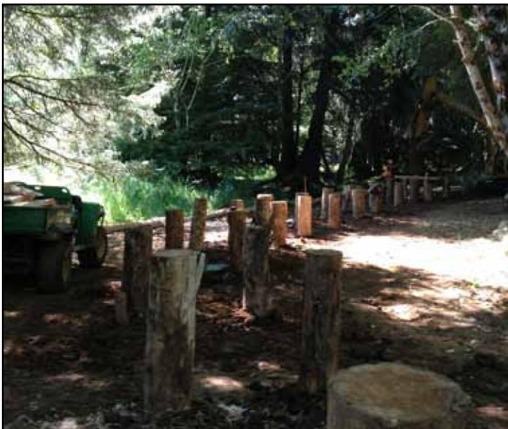
*Rows of pilings have replaced the western berm at Circle Creek, where a future boardwalk trail is planned.*
